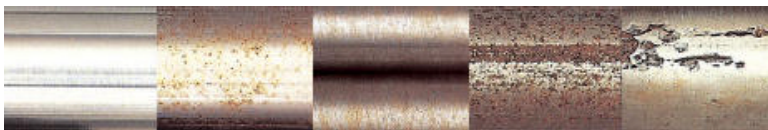
Example of stainless steel rust progression
