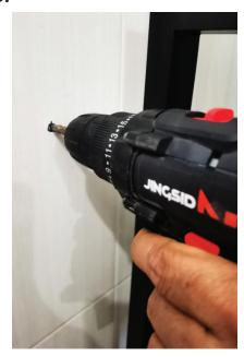
Drill pilot holes into the wall.
