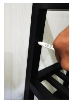
Locate the place where the sink will be installed. Use a pencil to identify where the mounting holes line up with the wall. This is when the adjusting feet should be made level.
